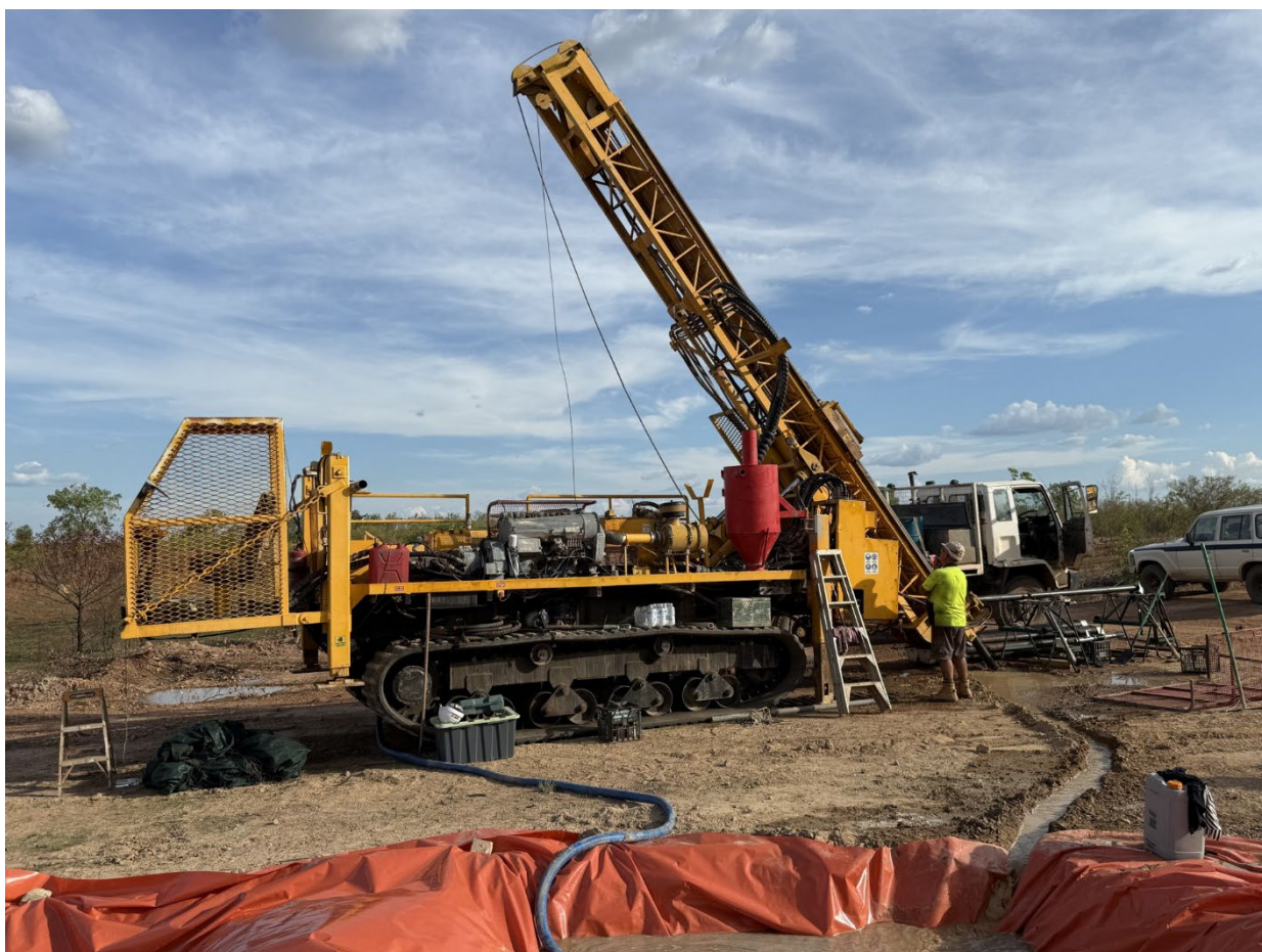
Figure 6: Johanssen Drill rig drilling WSP001
