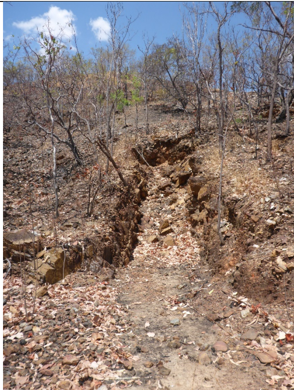
Looking south at Grants Prospect collapsed drive (NOTE: LW0014 taken up hill)
