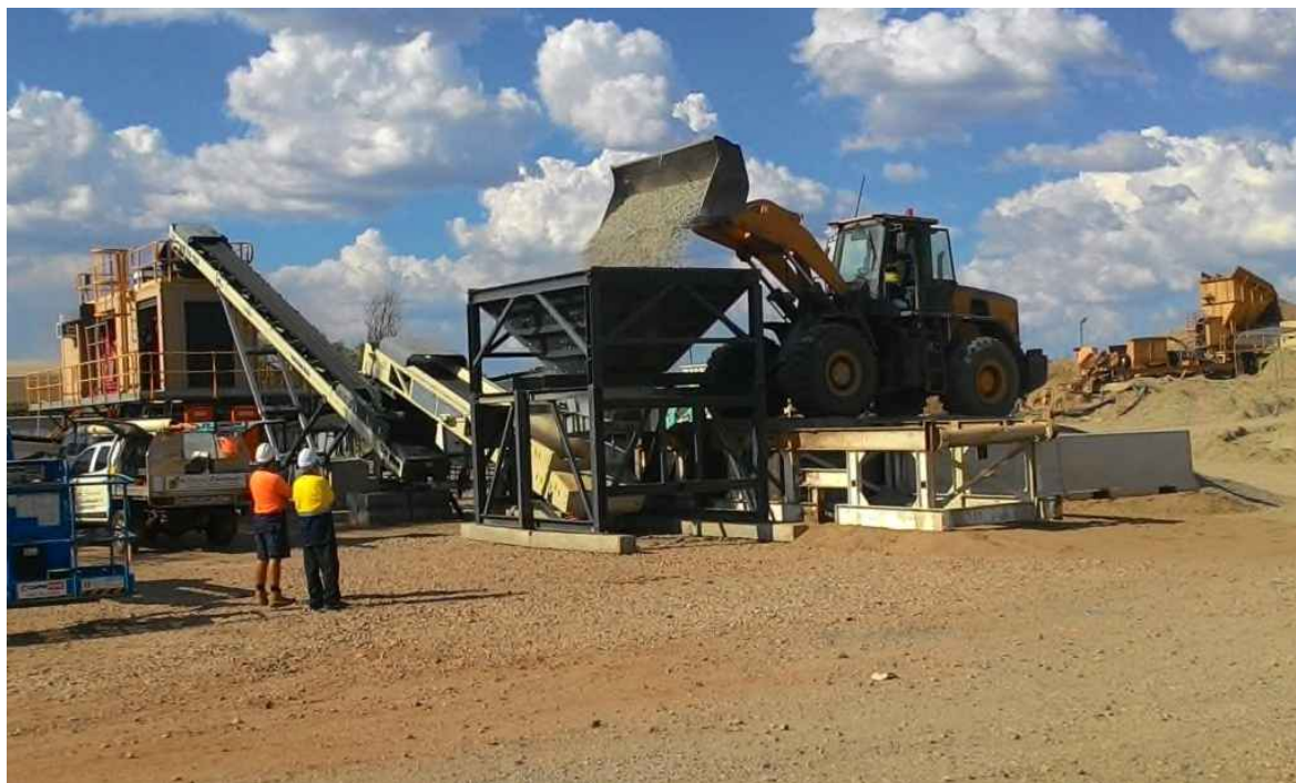
PHOTO 18: Batch feeding sized ore to TOMRA unit
