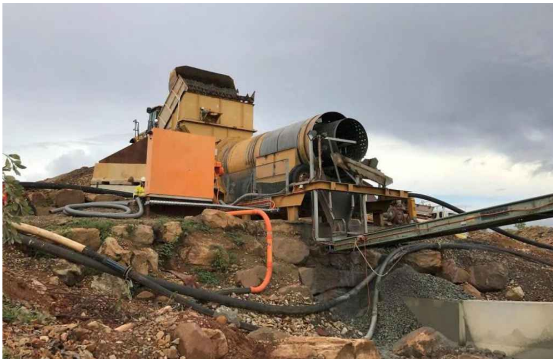
PHOTO 9: Scrubber commissioned in January 2017
