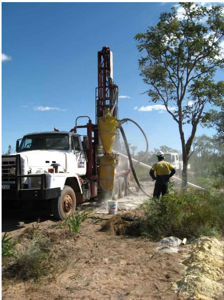
PHOTO 2: Orbit rig in action – drill spoil samples on right-hand-side
