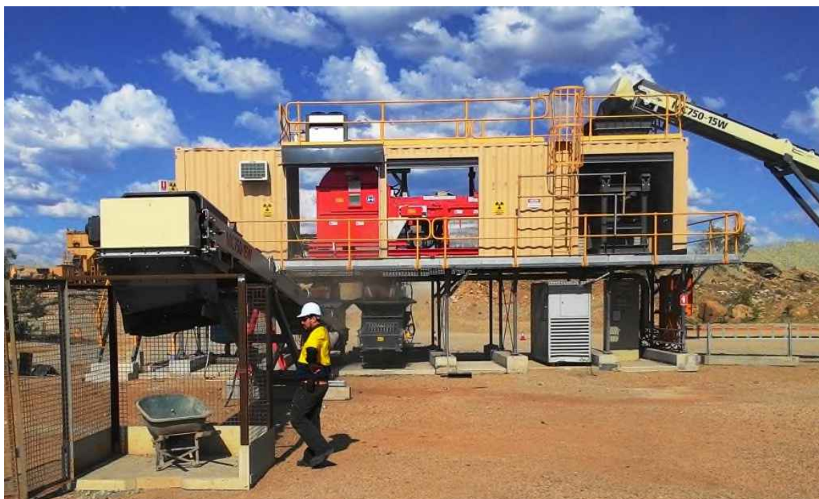
PHOTO 15: The Merlin TOMRA XRT is housed in a sea-container mounted on a raised platform When fully operational, concentrate from the TOMRA will be delivered to a hopper housed in a secured cage
