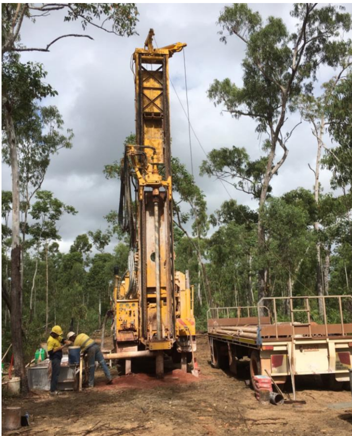
Plate 1: Groundwater Monitoring Bore Drilling
