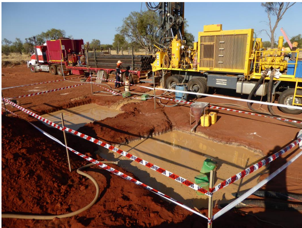
Stratigraphic drilling hole 2015/10P at Harts Range 489925E, 7461507N
