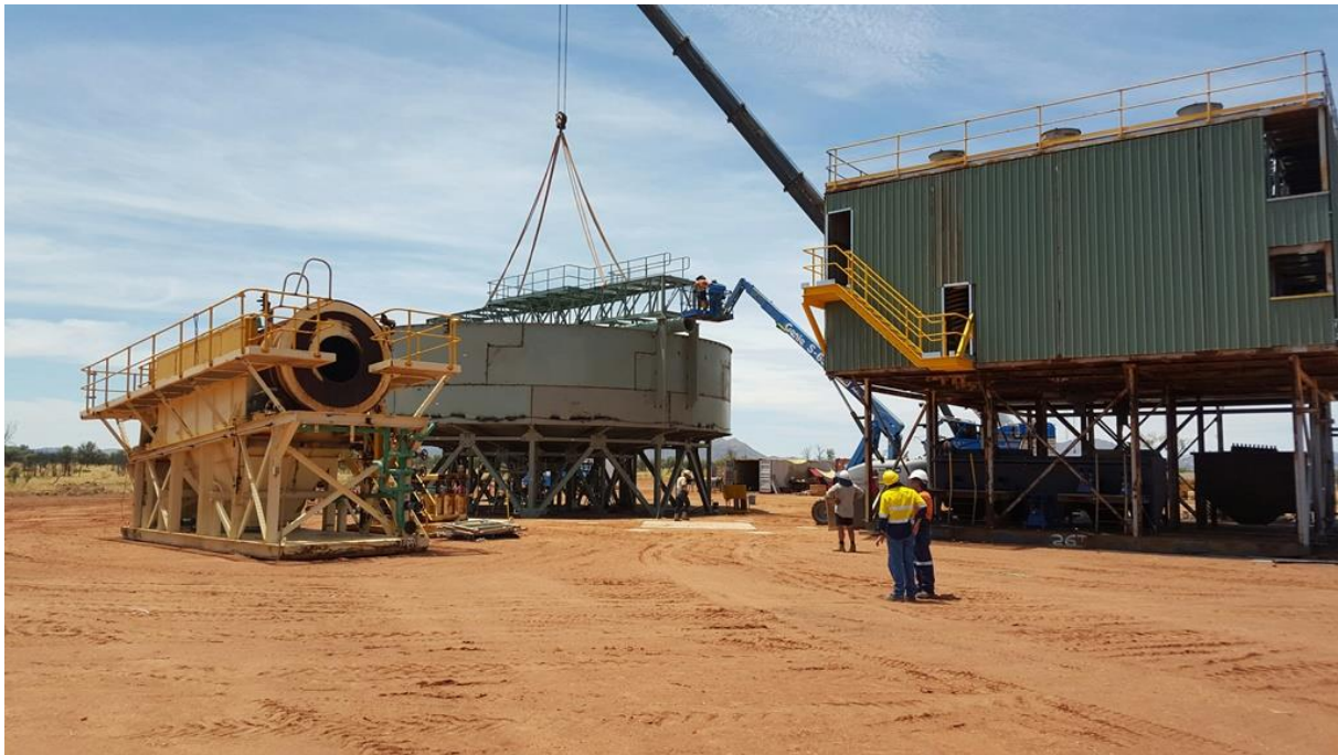
Construction of Plant at Spinifex Bore
