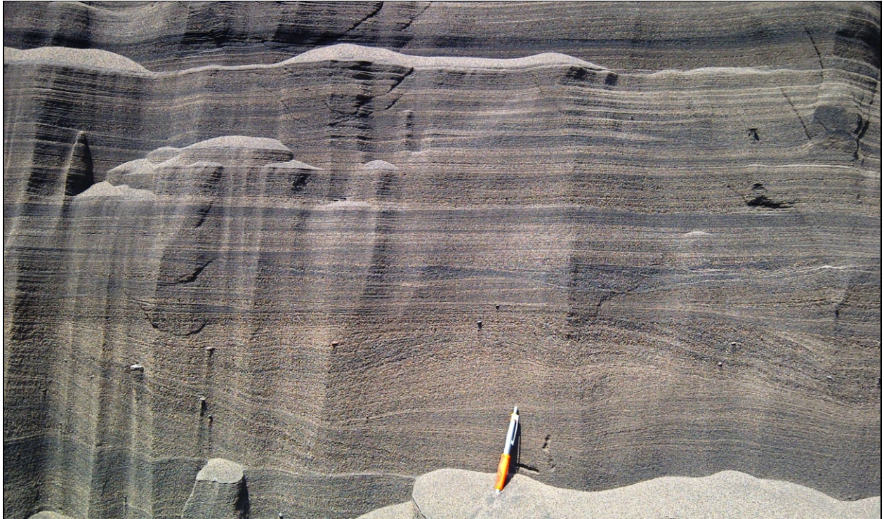
Figure 6 - C41 stockpile face close-up
