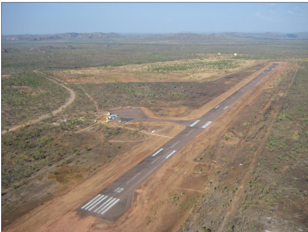
Figure 3: Aerial View of Nabarlek Camp and Airstrip
