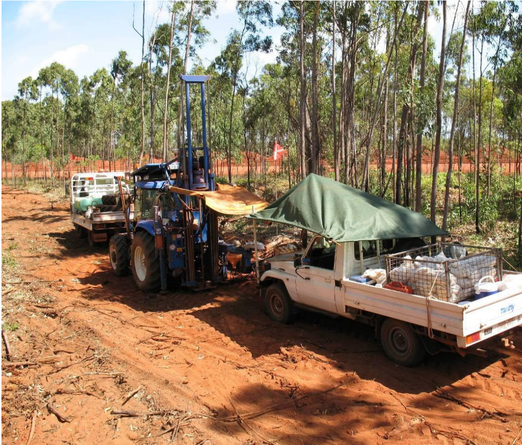
Figure 5-3 Tractor mounted vacuum drill rig and support vehicles. Source: Rio Tinto Alcan
