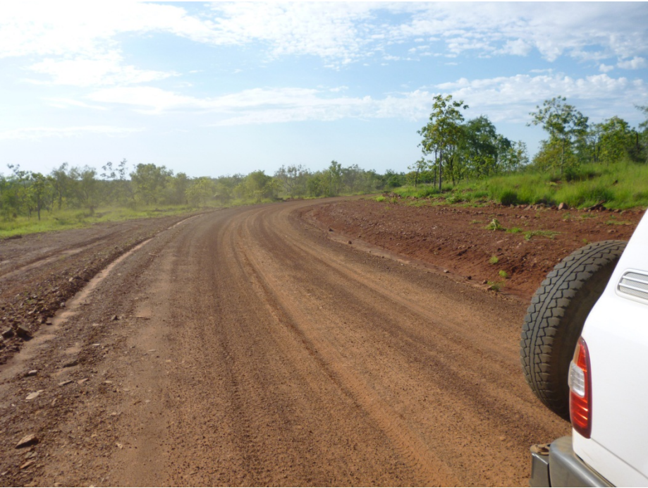
Additional view of 10km access road
