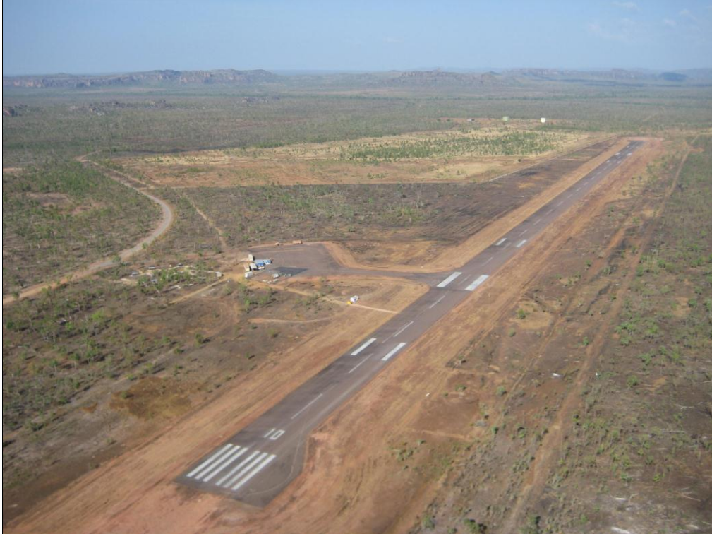
Figure 2: Aerial View of Nabarlek
