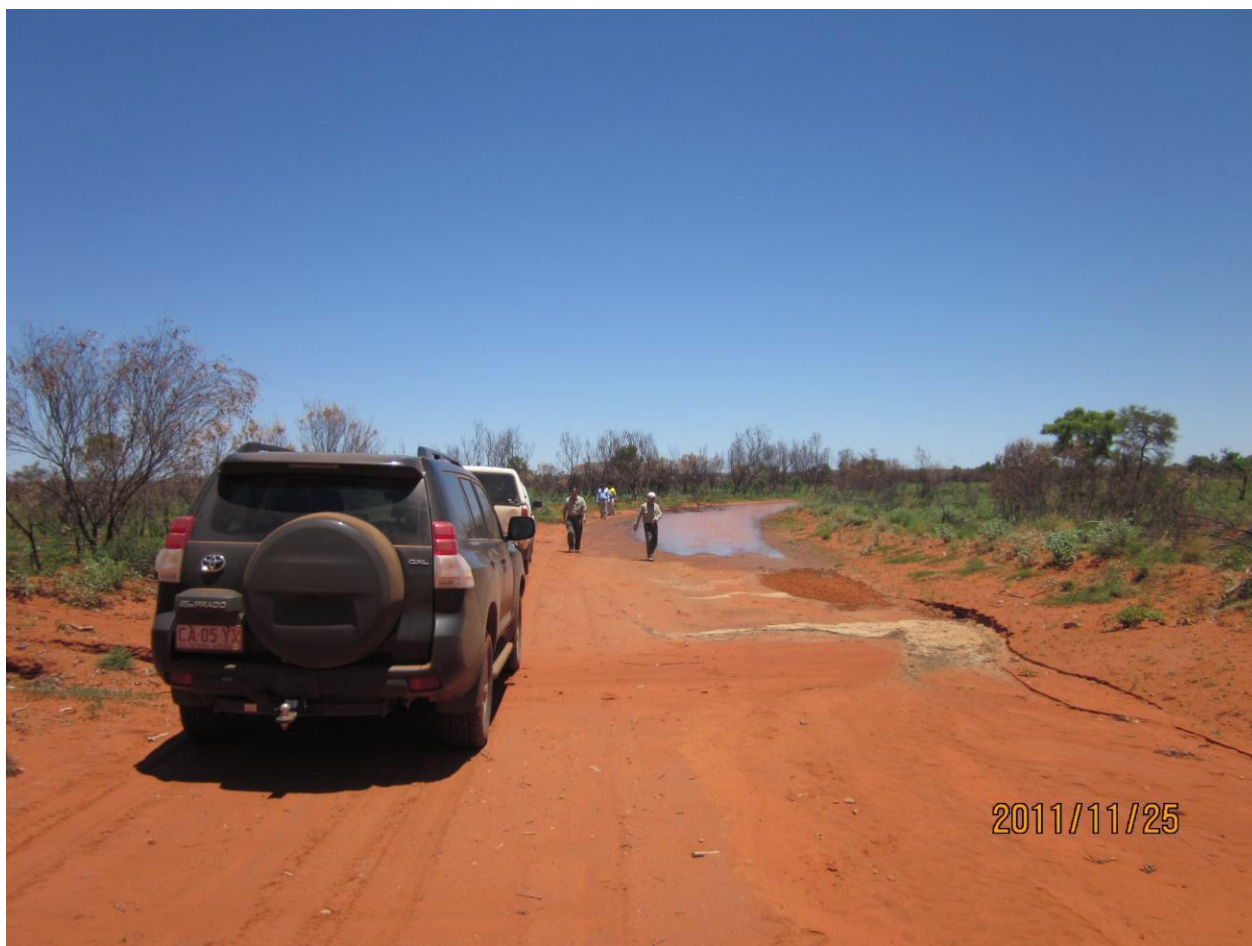
Photo1 Epenarra–old police station road surface gathered water (About 21 kilometres south of Epenarra)
