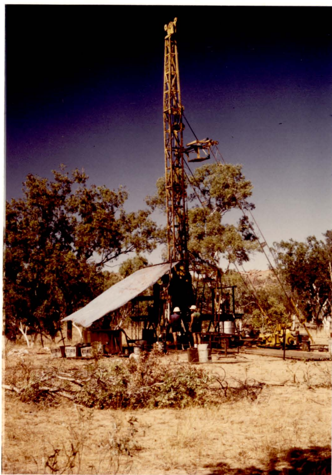
Plate 1-3. Long year 44 Diamond Coring Rig on site at Corehole 82-7: Jumping Wallaby No. 1. This rig disassembled into sixteen segments and was shuttled between coresites by a Bell 206-B Jet Ranger III helicopter. The heaviest component of the rig is the gear box, weighing on the order of 1300 pounds.
