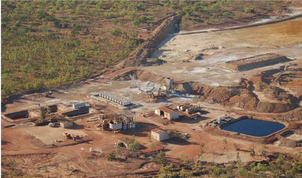
Figure 2: Redbank Infrastructure on ERL94, July 2009
