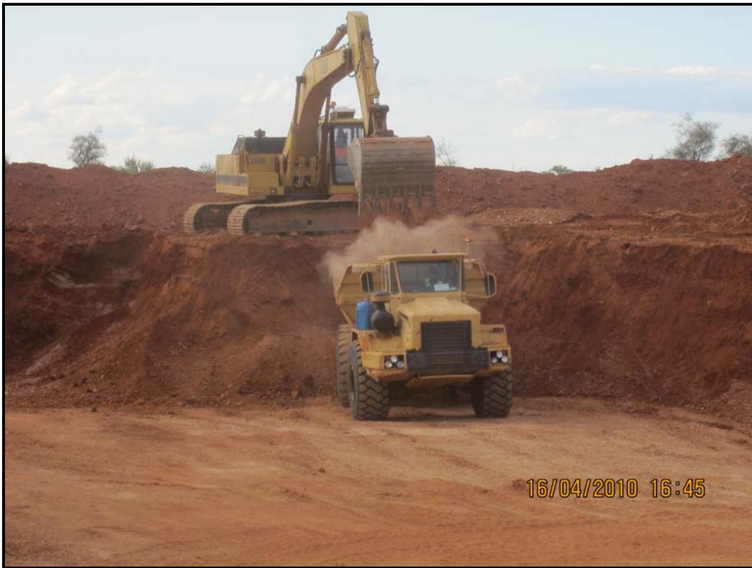
Photograph 3 – Removing gravel for road construction from the gravel borrow pit.
