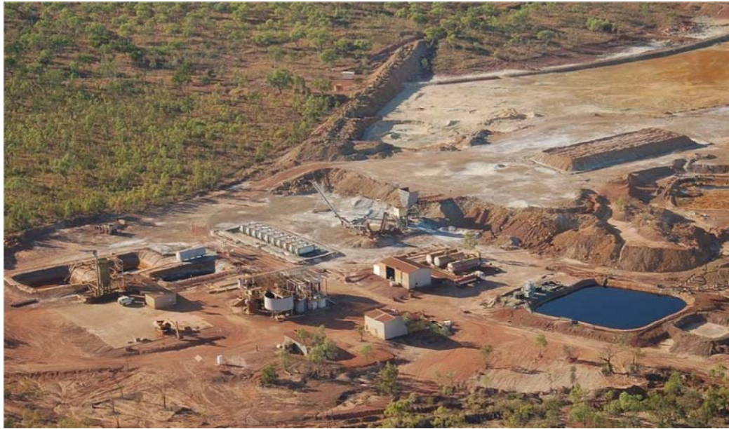
Figure 2: Redbank Infrastructure on ERL94, July 2010
