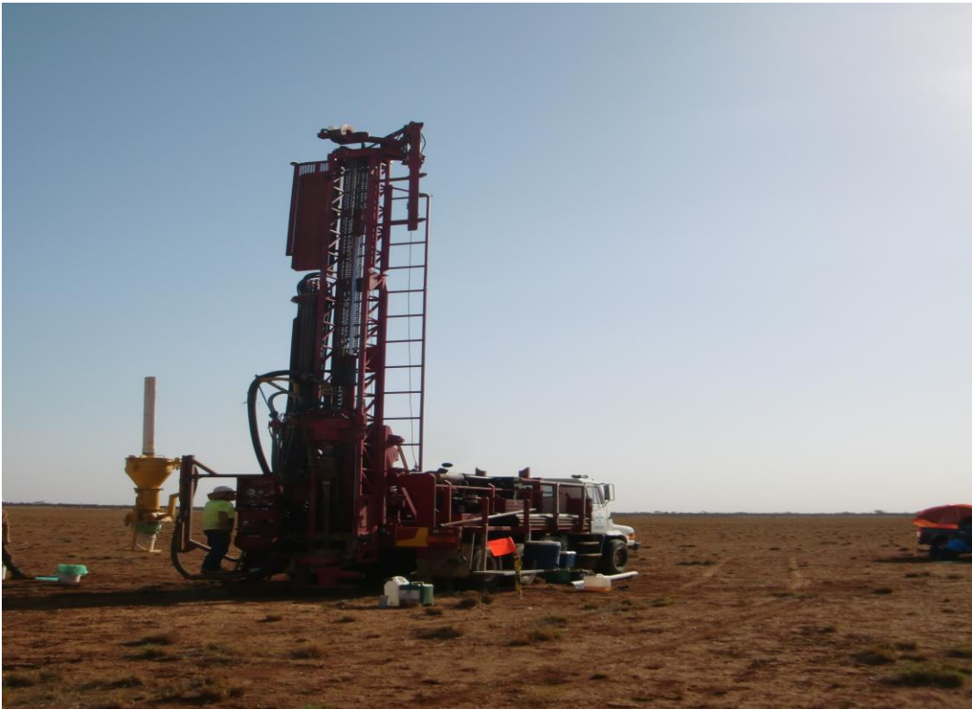
Figure 5: Schramm 450 drilling rig mounted on custom built 6x6 carrier
