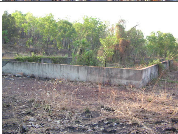
Concrete foundation- Helene pit offices
