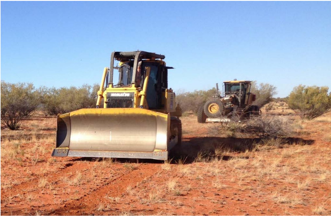
Photograph 4: Dozer with Grader following up
