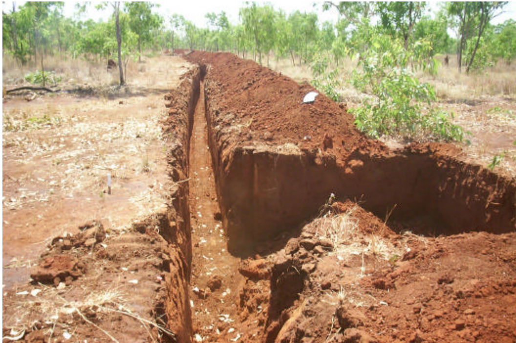
Buka Trench 1 : Following excavation
