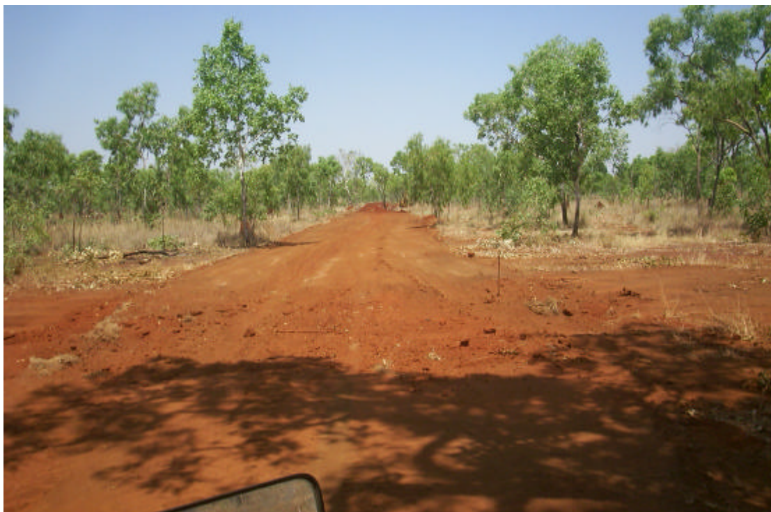
Buka Trench 1 : Infilled after completion of sampling
