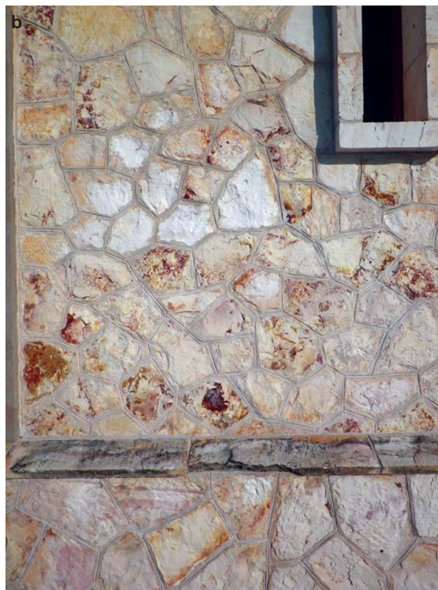
Figure 40.14. (a) Porcellanite block work in St Mary's Cathedral, Darwin. (b) Detail of block work in bell tower of St Mary's Cathedral.
