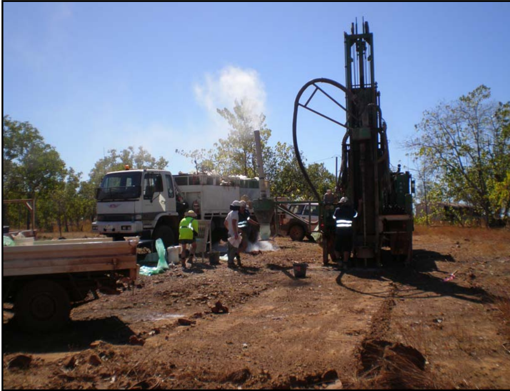
Photo 3; Drill pad 3x loader scrapings wide and twice drill rig length.
