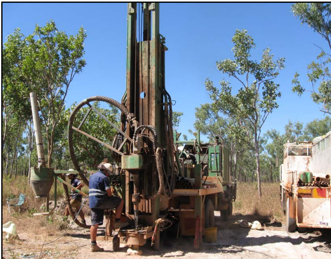
Photo 4; Drill pad location selected between trees
