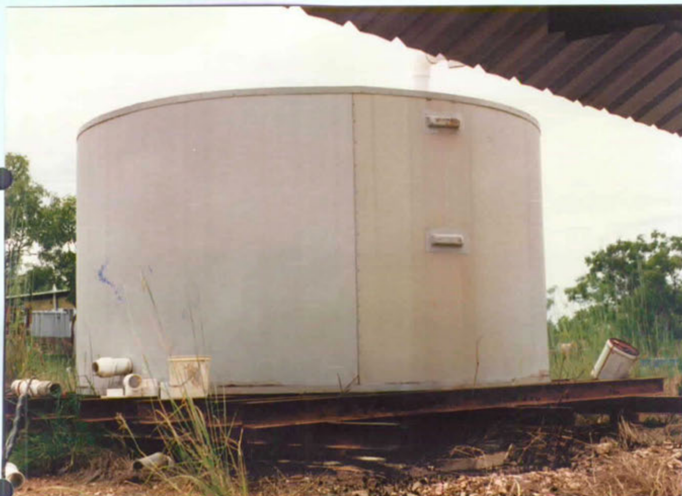
DIRTY PROCESS WATER TANK IN POSITION.
