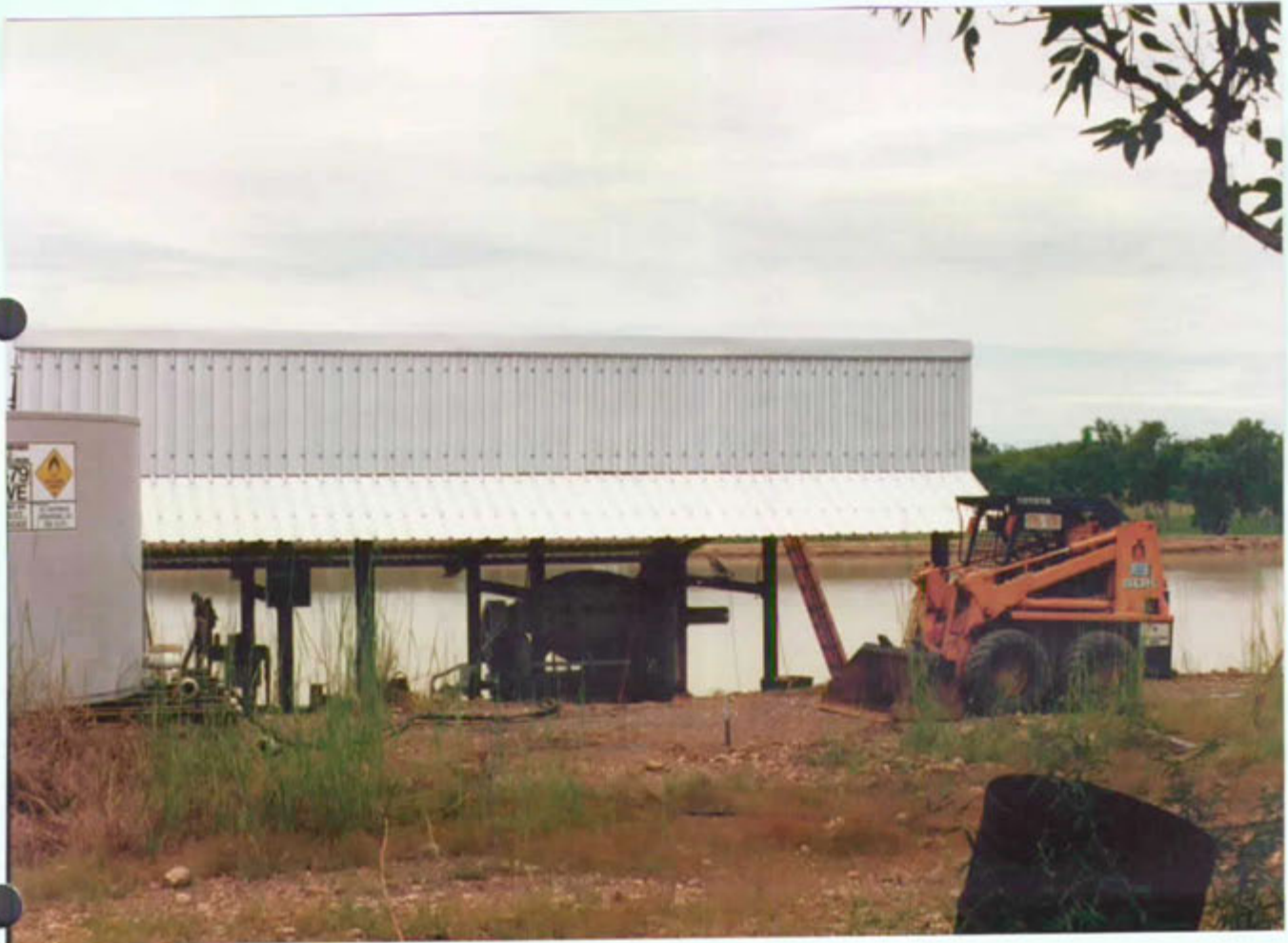
PROCESS PLANT BUILDING & PROCESS WATER DAM IN THE BACKGROUND.
