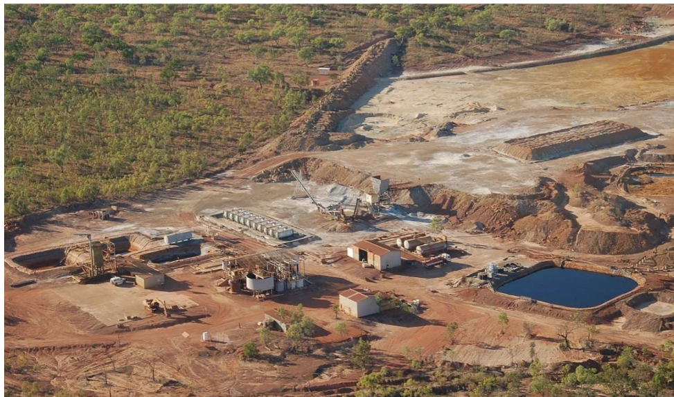
Figure 2: Redbank Infrastructure on ERL94, July 2011
