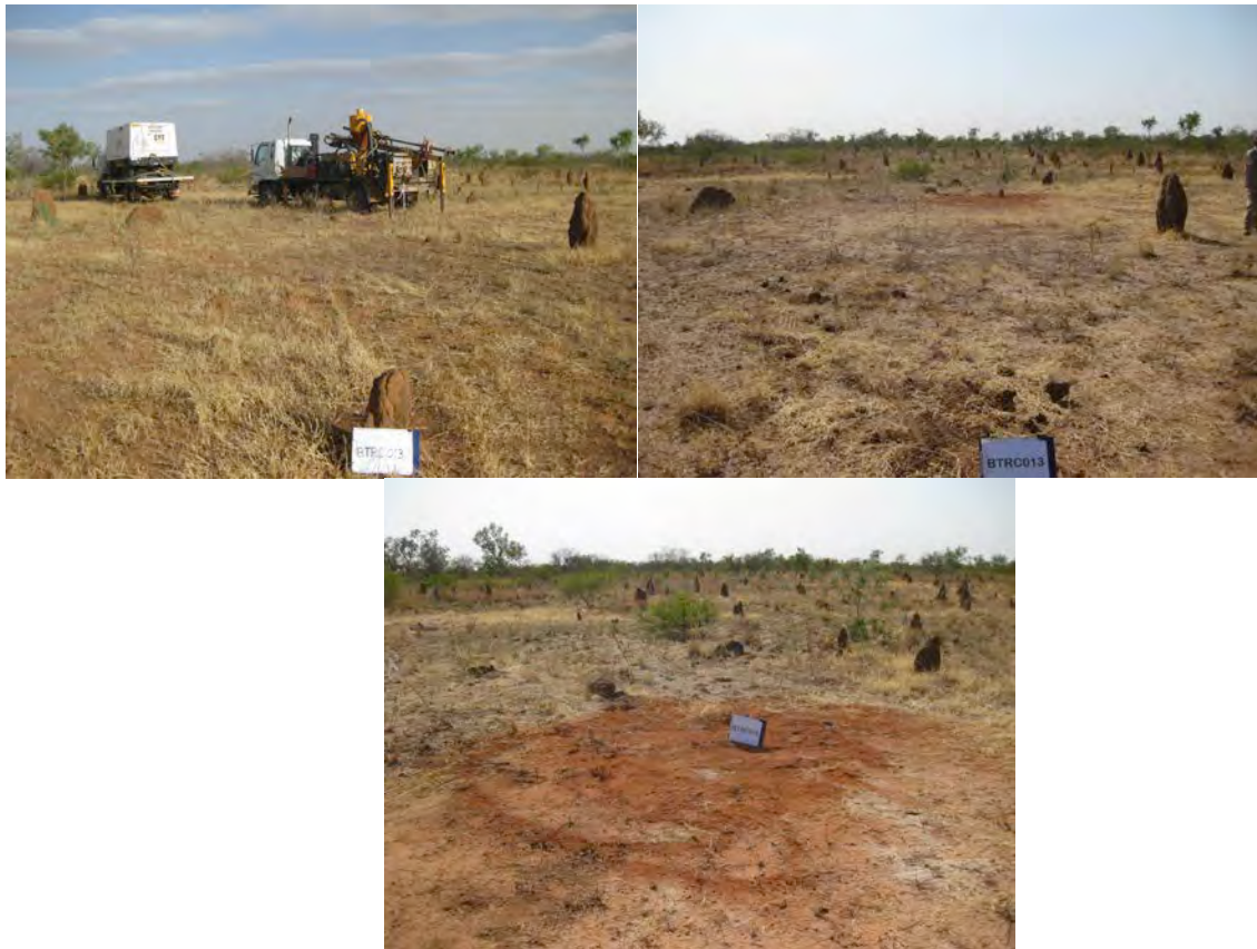
Figure 5: Drillhole BTRC013 rehabilitation. Site before and after, and final collar as left.
