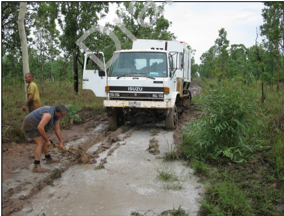
Photo 10: Compressor truck bogged on Hayes Creek access track
