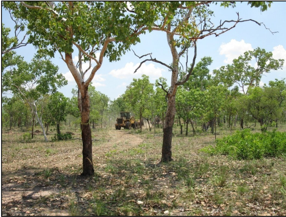
Photo 1: Establishing drill site access at Tennyson's, south of Edith River
