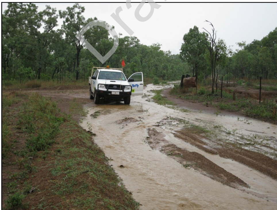
Photo 8: Stormwater runoff on drill access track
