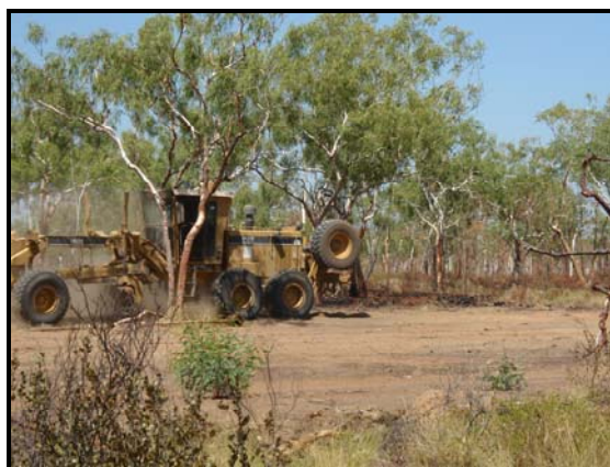
Plate 2 Drill site CHRCD002-Grader completing rehabilitation
