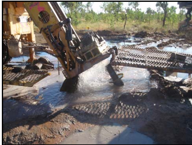
Plate 11 Flowing bore at CHRCD004 (app. 30,000L/hr)
