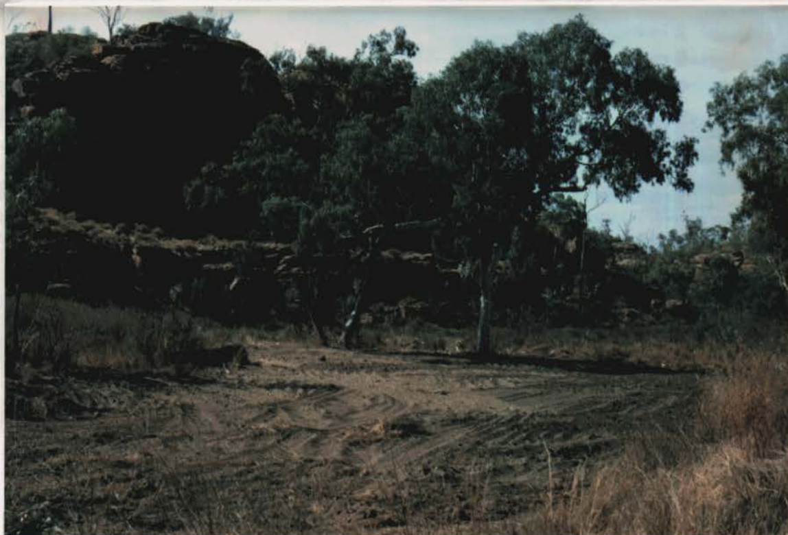
PHOTO 5 View looking southeast at site E1C, showing levelled and filled mullock/costean site, contoured with topsoil.
