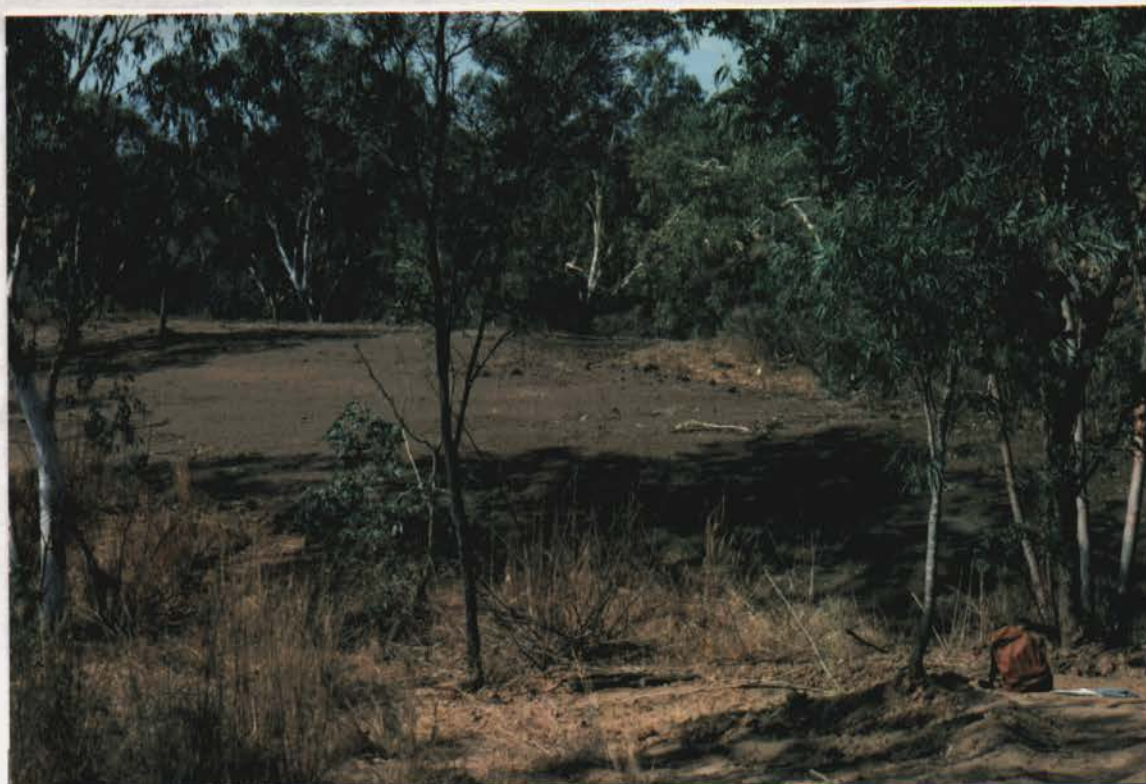
PHOTO 2 View looking southwest at site E1E showing levelled and filled mullock/costean site, now contoured with topsoil.
