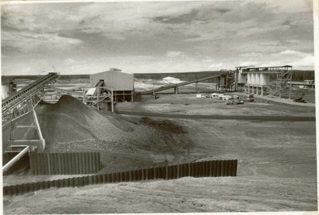
Concentrating plant from primary crushing station. Surge stockpile at left, product bins at right.
