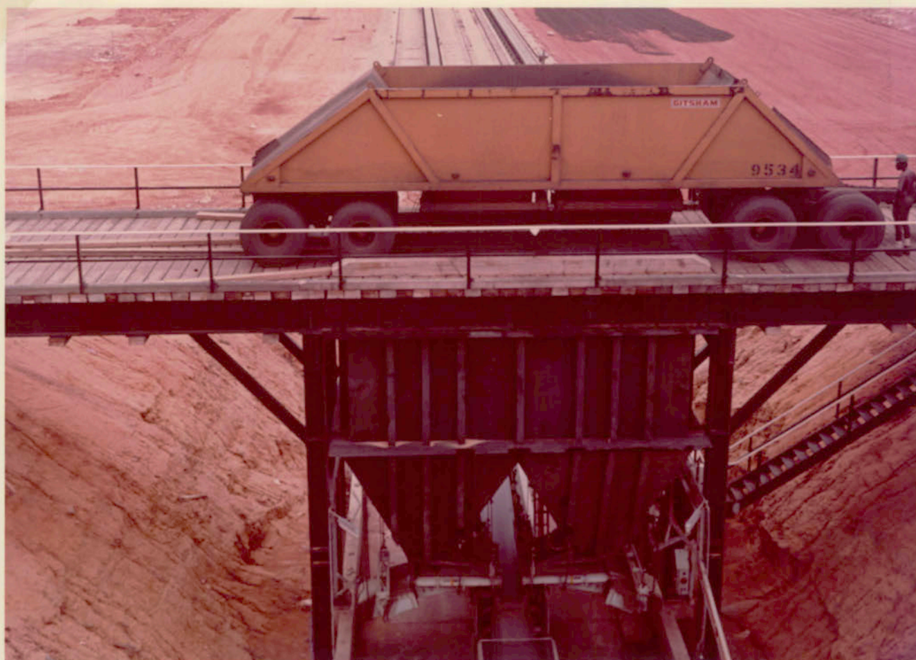
45 ton trailer discharging into new hopper at shiploading stockpile area.
