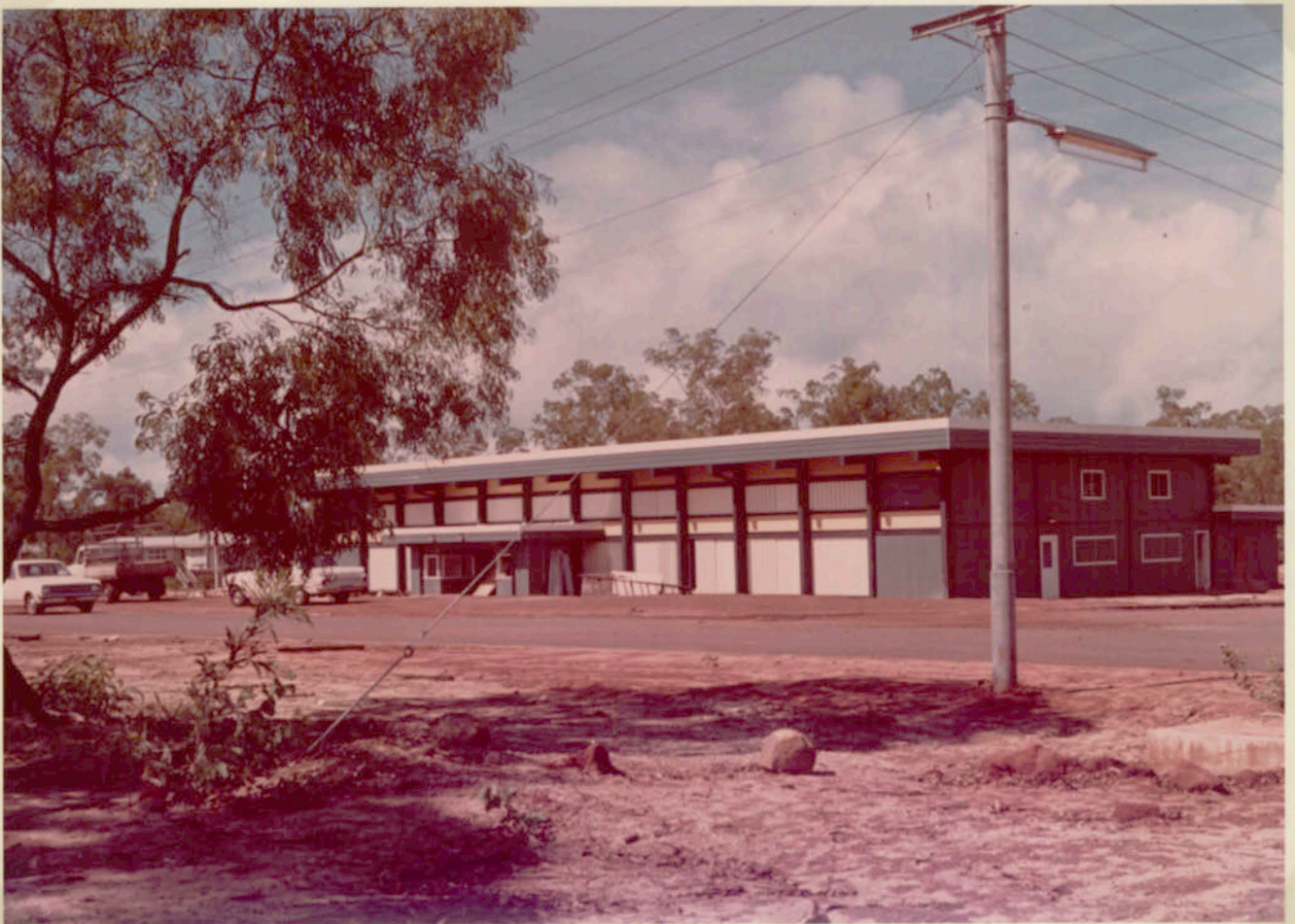
New Community Hall in township.
