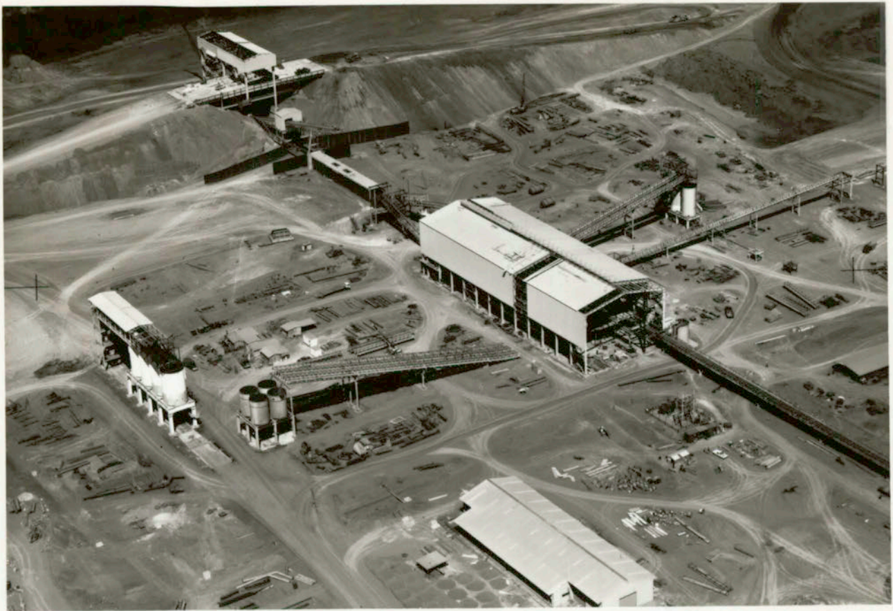
View of concentrator plant (centre) taken in August 1971, with primary crushing station at upper, product bins at left and store at lower.
