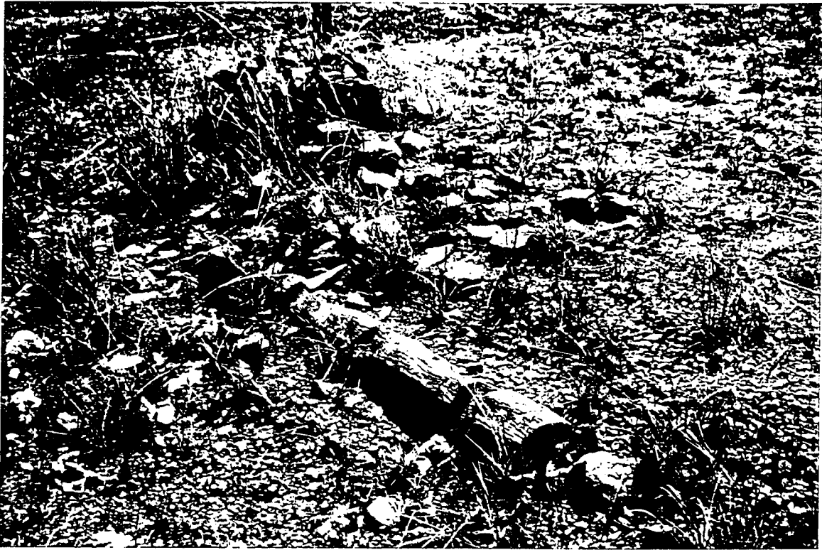
PLATE FIVE - Notched log at temple site entry, between concrete post bases.
