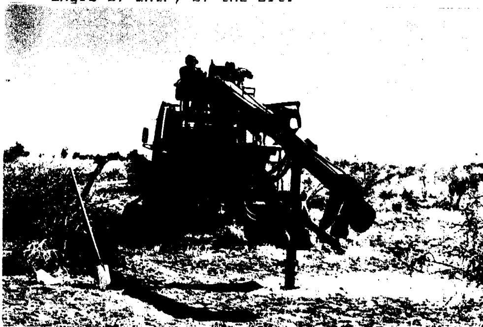
Photo 4. Drill completing a hole to full length of Kelly bar.
