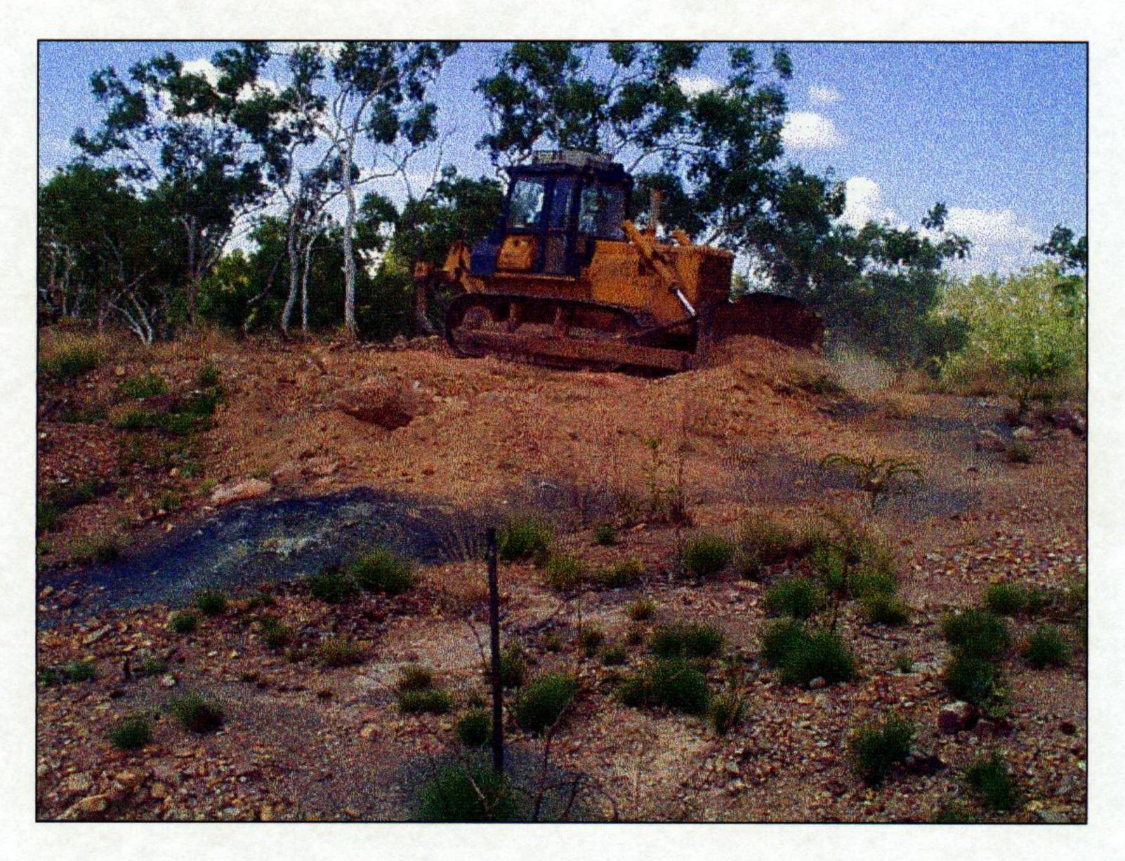
Figure 14 Redistributing Ripped Soil and Clay on Drill Site
