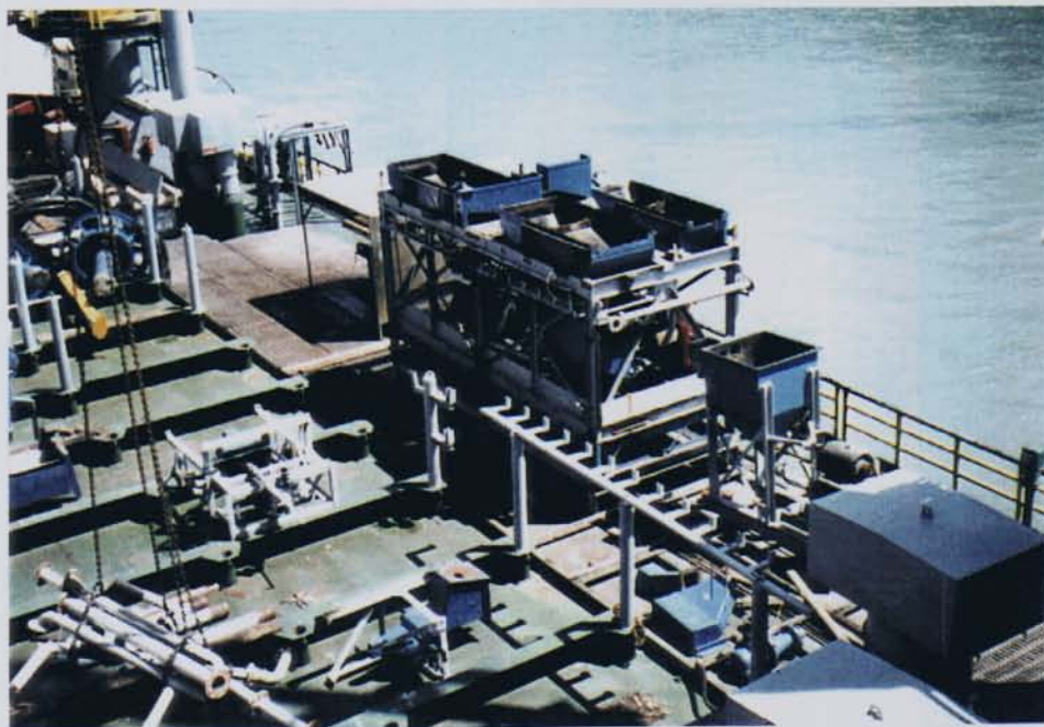
Figure 6-1 Installation of the Dense Media Separation (DMS) plant.
