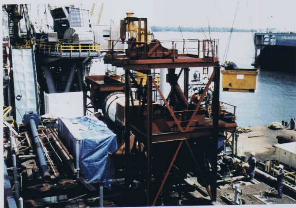
Figure 6-2 Installation of the "triple deck" onto the top of the process plant.
