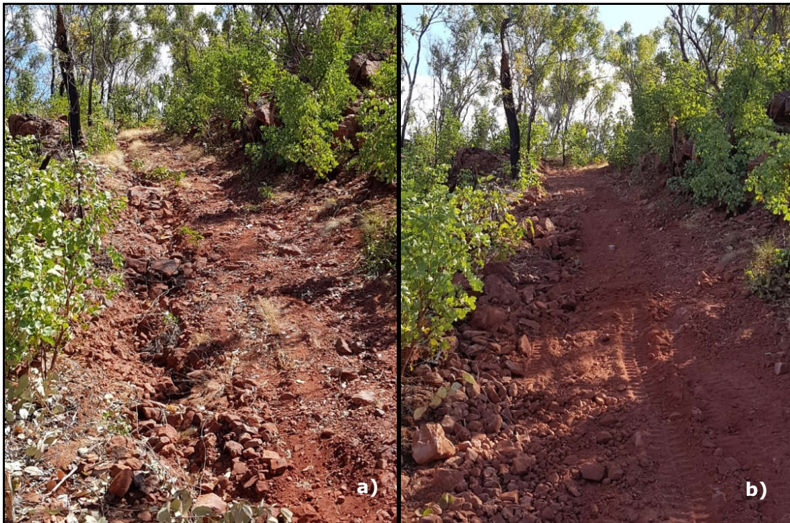
Plate 2: Track up Legune Hill, a) BEFORE, b) AFTER, remediation
