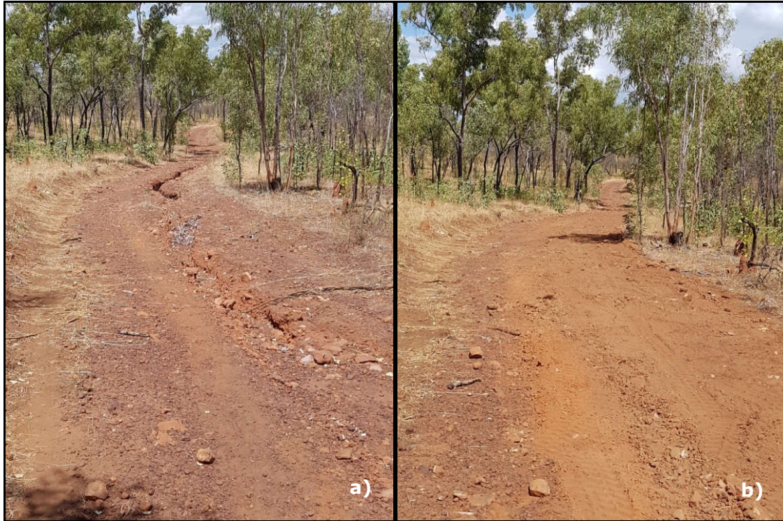
Plate 1: Track heading north from Legune Road, a) BEFORE, b) AFTER, remediation.
