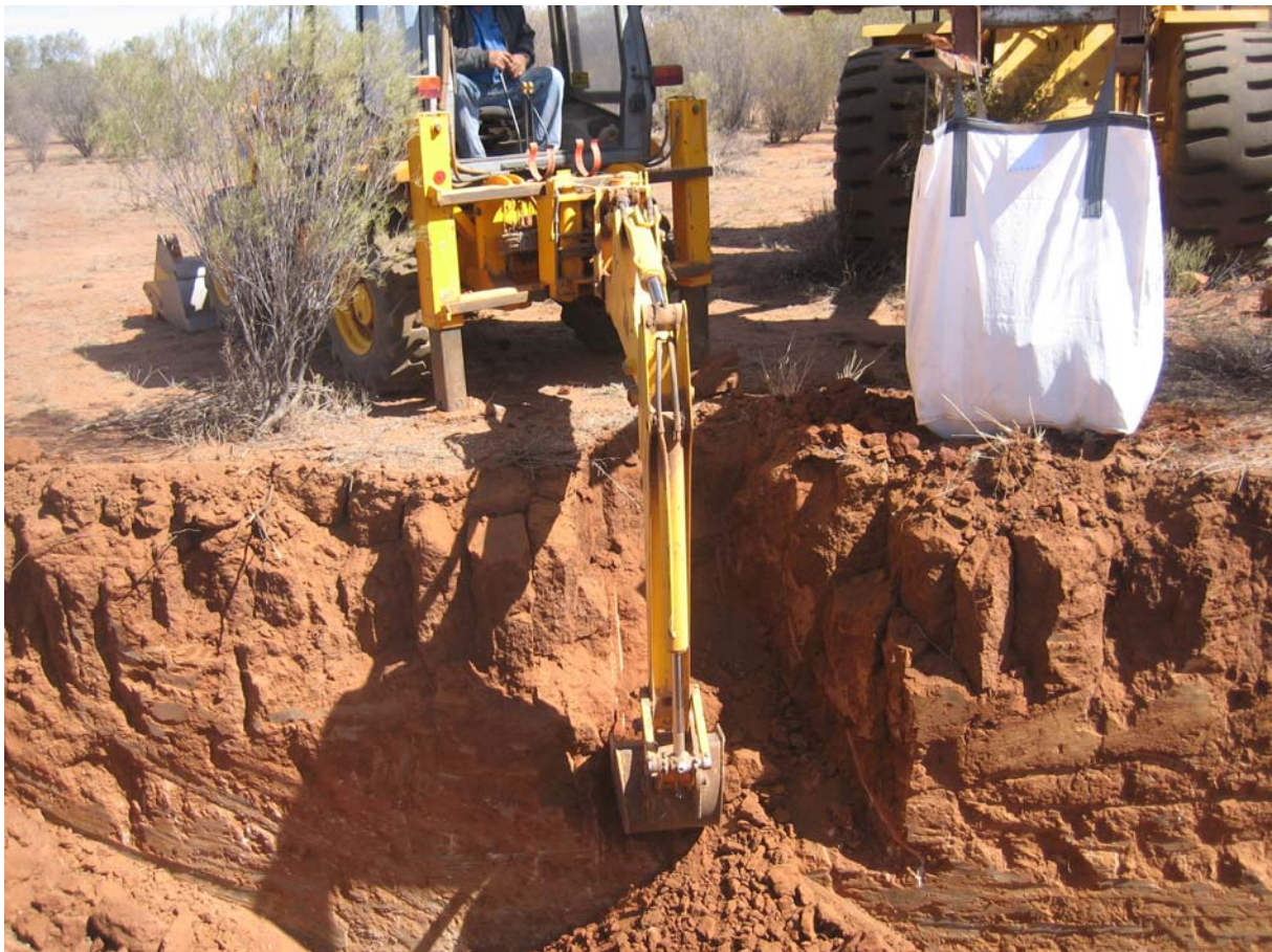
Figure 2 Backhoe and Payloader used in 2nd programme showing floodplain
